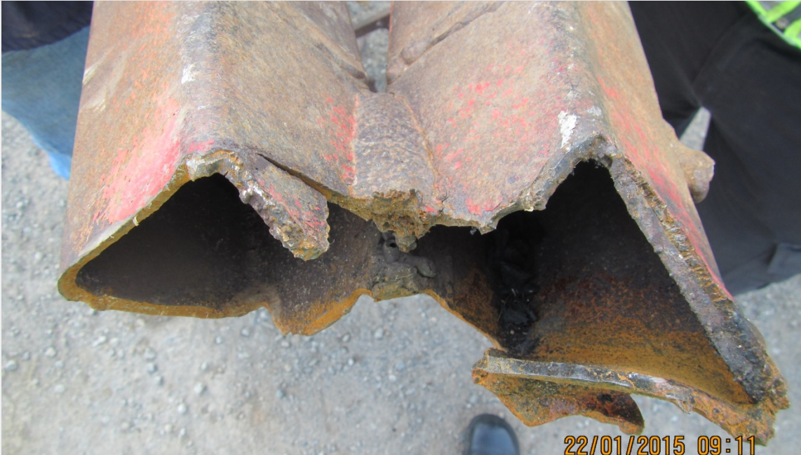
Head of draw bar broken away Old age , metal fatigue and poor welding
